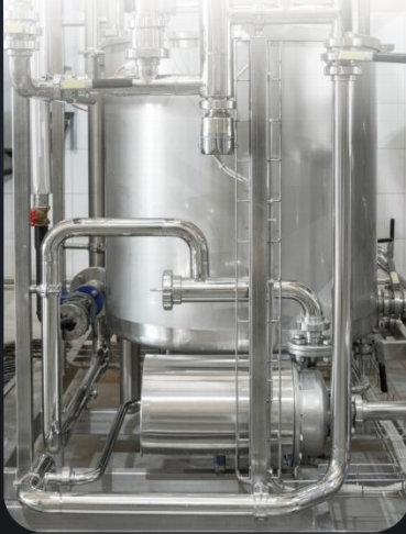
Mechanical and electrical circulating water equipment
